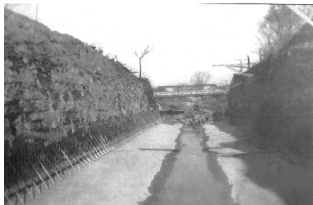
Pictured above: Construction of the locks during the late 1930's.
